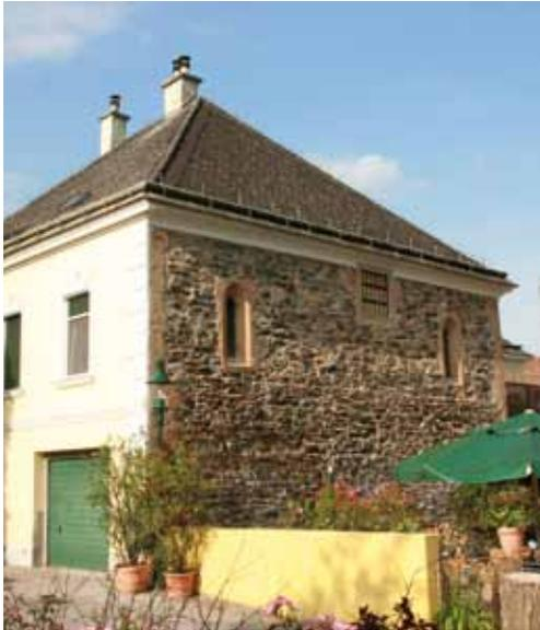
The medieval synagogue lies on the right as one enters the narrow Fischergasse. It dates from the 13th century and consists of Gothic dry stone walls with dressed cornerstones. Two Gothic jambs stem from the construction period. An addition was added to the building on the north side in the 16th century; the current façade was built in 1900.
